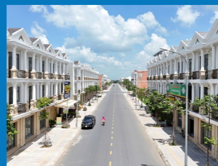
D7 ROAD PROJECT
